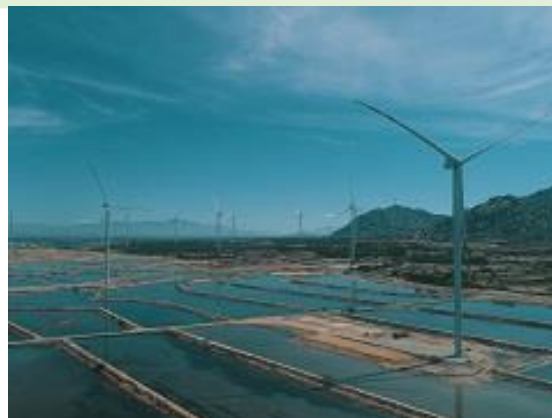
Construction of wind power plants in Vietnam
