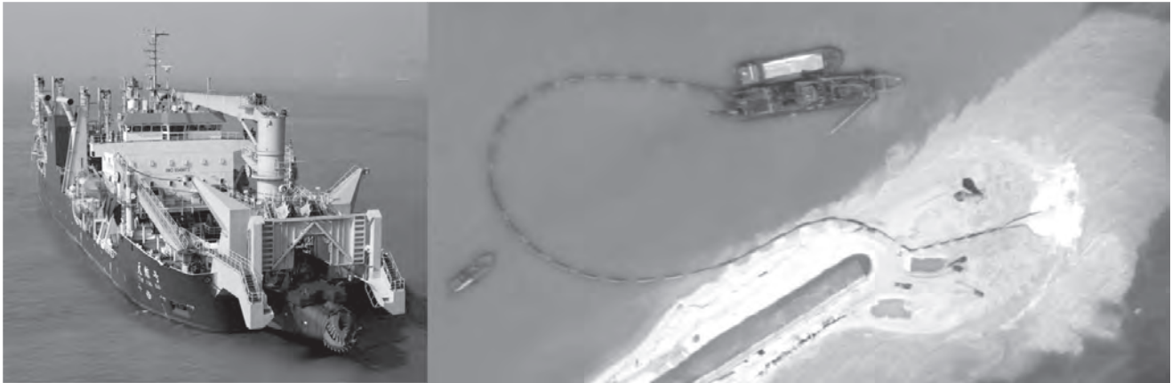
Figure 10.4. Dredging and Island Construction
